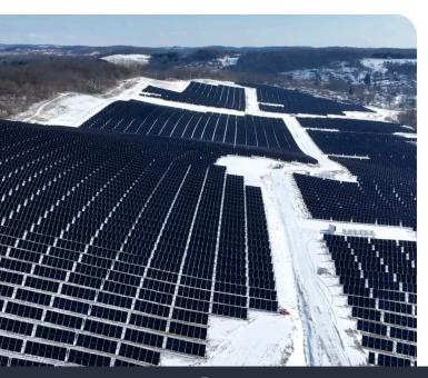
Unlike traditional systems that would require extensive grading to achieve 5% to 8% slope tolerances, Nevados' ATT allowed for Ampliform to reduce grading from the existing 30% slopes down to their preference of only 20%. The ATT minimized soil disruption and reduced project costs, while working with the natural landscape to avoid unnecessary risk.
