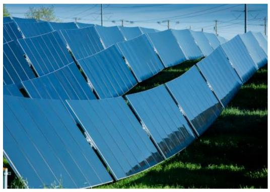
The Nevados TRACE™ All Terrain Tracker®, "Best in Show" in the Large-Scale category of Solar Power World's 2024 Top Products contest, tackles steep and undulating terrain of up to a market-leading 37% slope, and undulating capability of 26% at every post, eliminating costly and environmentally destructive grading.
