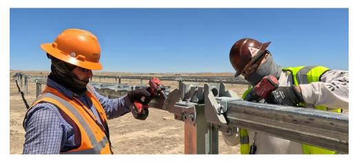
Milwaukee Tool's new M18 FUEL<sup>™</sup> Controlled Torque Impact Wrench with TORQUE-SENSE<sup>™</sup>, in tests on Nevados' TRACE<sup>™</sup> All Terrain Tracker<sup>®</sup>, demonstrated it can tighten bolts over three times faster. Photo credit: Eclipse-M
