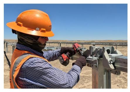
Milwaukee added machine learning to its Controlled Torque Impact Wrenches so they self-adjust to conditions as they apply the correct torque to a bolt. Photo credit: Eclipse-M
