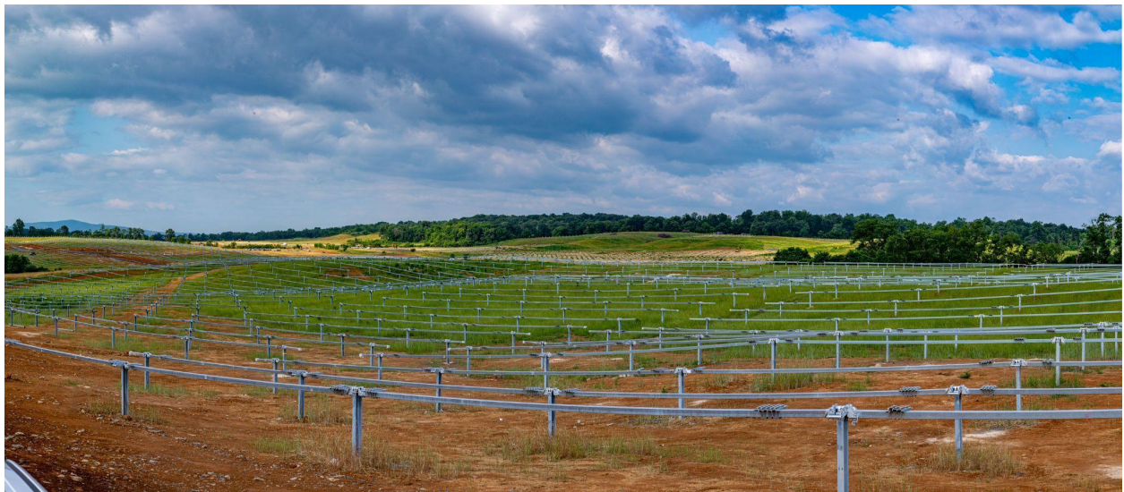
Nevados' All-Terrain Tracker in use on the new 170 MW solar farm.
